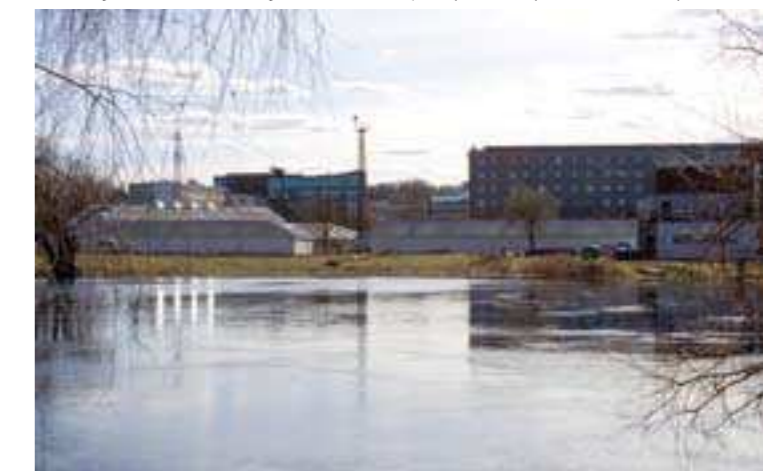
The back wall of the open market that blocks the embankment
